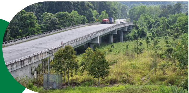
Figure 32: Viaduct in Gerik, Perak (CFS 1 PL 2: Temenggor FR – Royal Belum State Park) completed in 2015 that cost RM25 million
